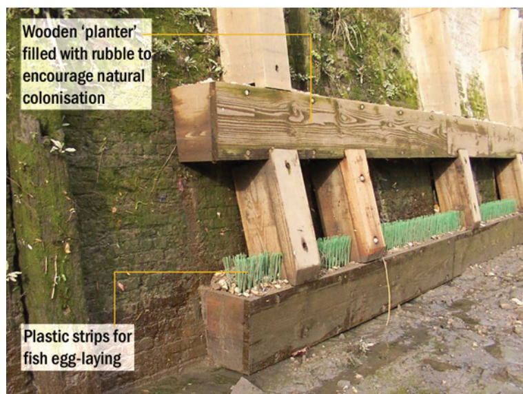
Deptford Creek, London: Timbering to river wall
