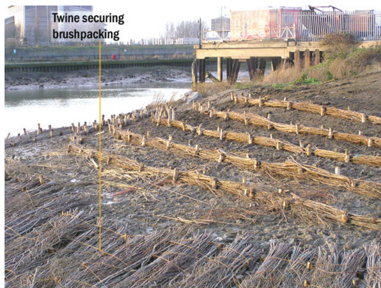
Barking Creek at Barking Barrier: Fixing detail of brushpacking
