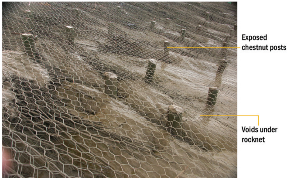
Monk Bretton site near bridge: Rocknet and fascine installation showing size of drainage rivulet
