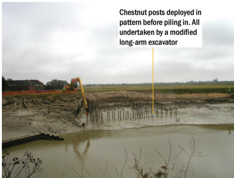
Monk Bretton site near bridge: Installation of posts for fascines
